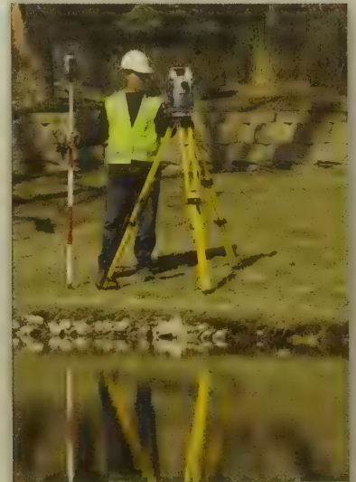
Surveying (Exercise 39, p. 311)
